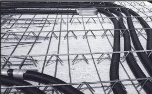
If flexible ducts are inserted into ceilings with fire protection requirements, minimum ceiling thicknesses and/or minimum thicknesses above and below the inserted parts must be taken into account. The precise installation situation should be clarified with the local site engineer based on the fire protection concept for the building. Also refer to DIN 4102-4 3.4 Tables 9 and 10.
