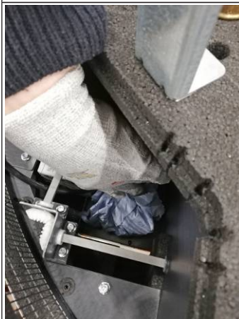
Fig. 36: Cleaning the pump sump
