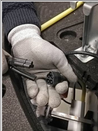
Fig. 35: Loosening the cable
